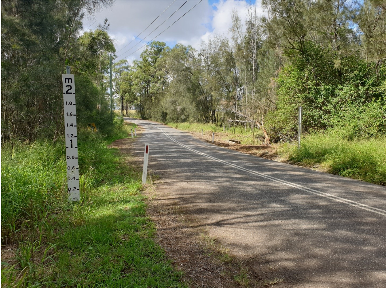
Photo 6: Existing flood depth indicators on Gillards Road near 600 mm pipe culvert, looking east
