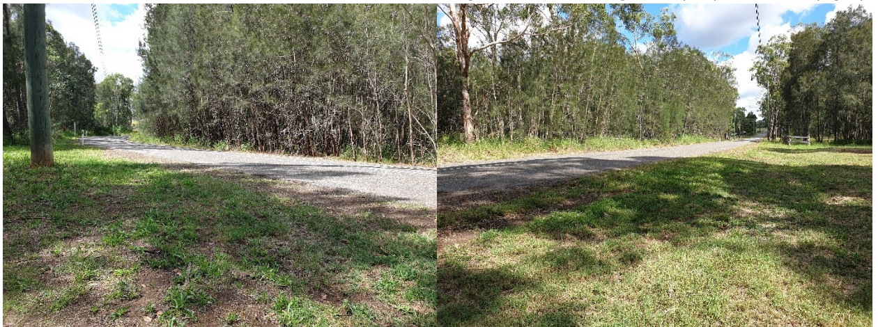
Photo 3: Lowpoint of Gillards Road between existing culverts, looking east (left) and west (right)
