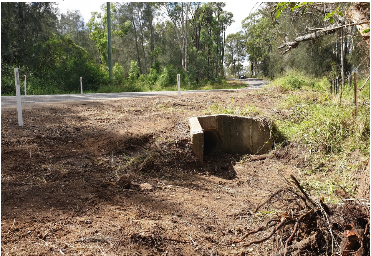
Photo 1: Existing 600 mm pipe (eastern culvert) at Gillards Road (upstream)
