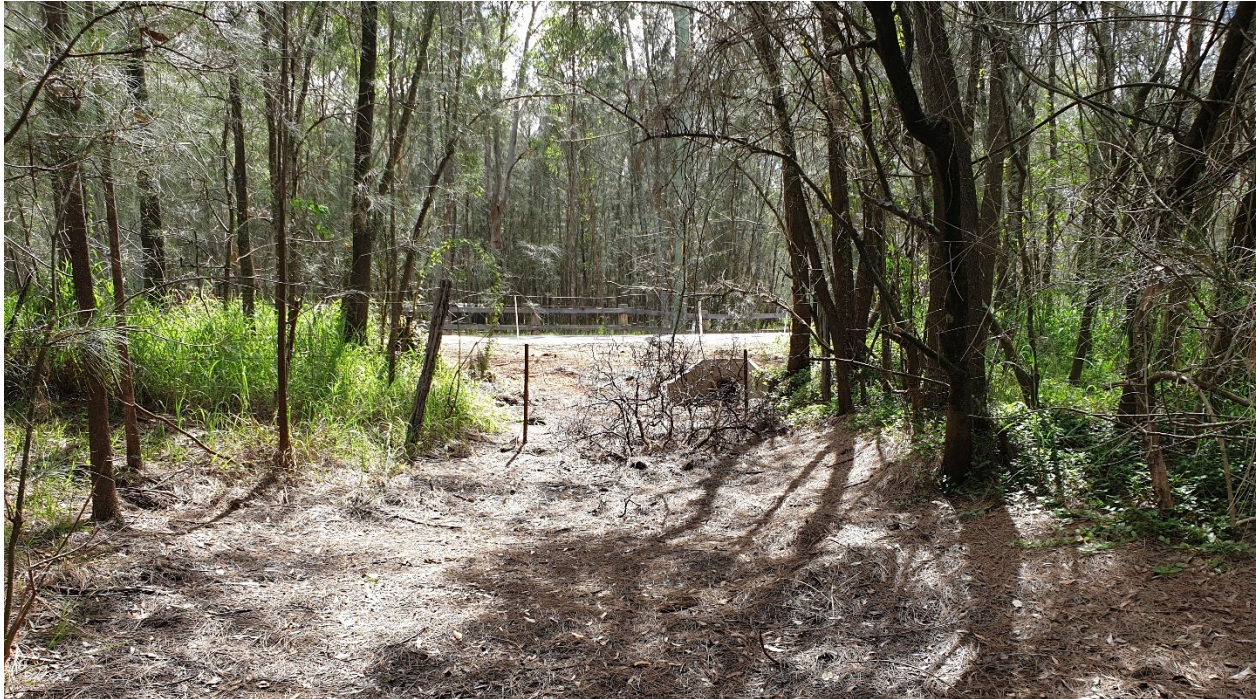
Photo 2: Existing 450 mm pipe (western culvert) at Gillards Road
