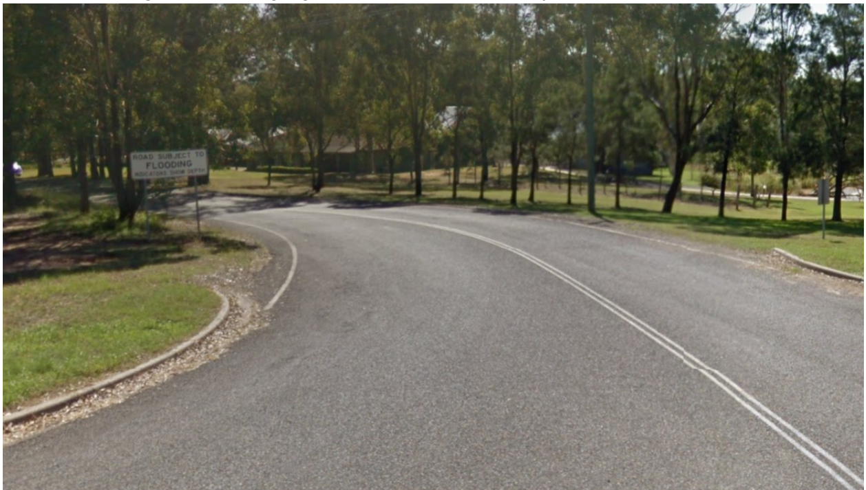
Photo 5: Existing flood warning sign on Gillards Road at entry from McDonalds Road
